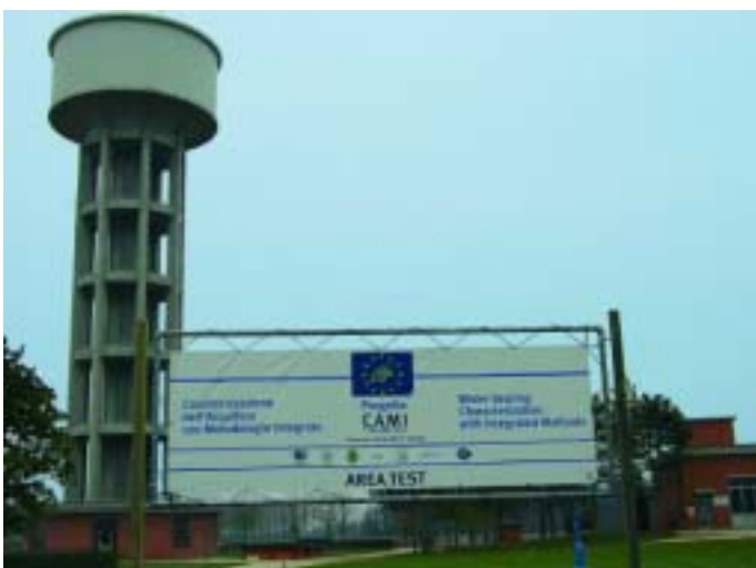
Piezometric tower – ABL (Torrate di Chions).
